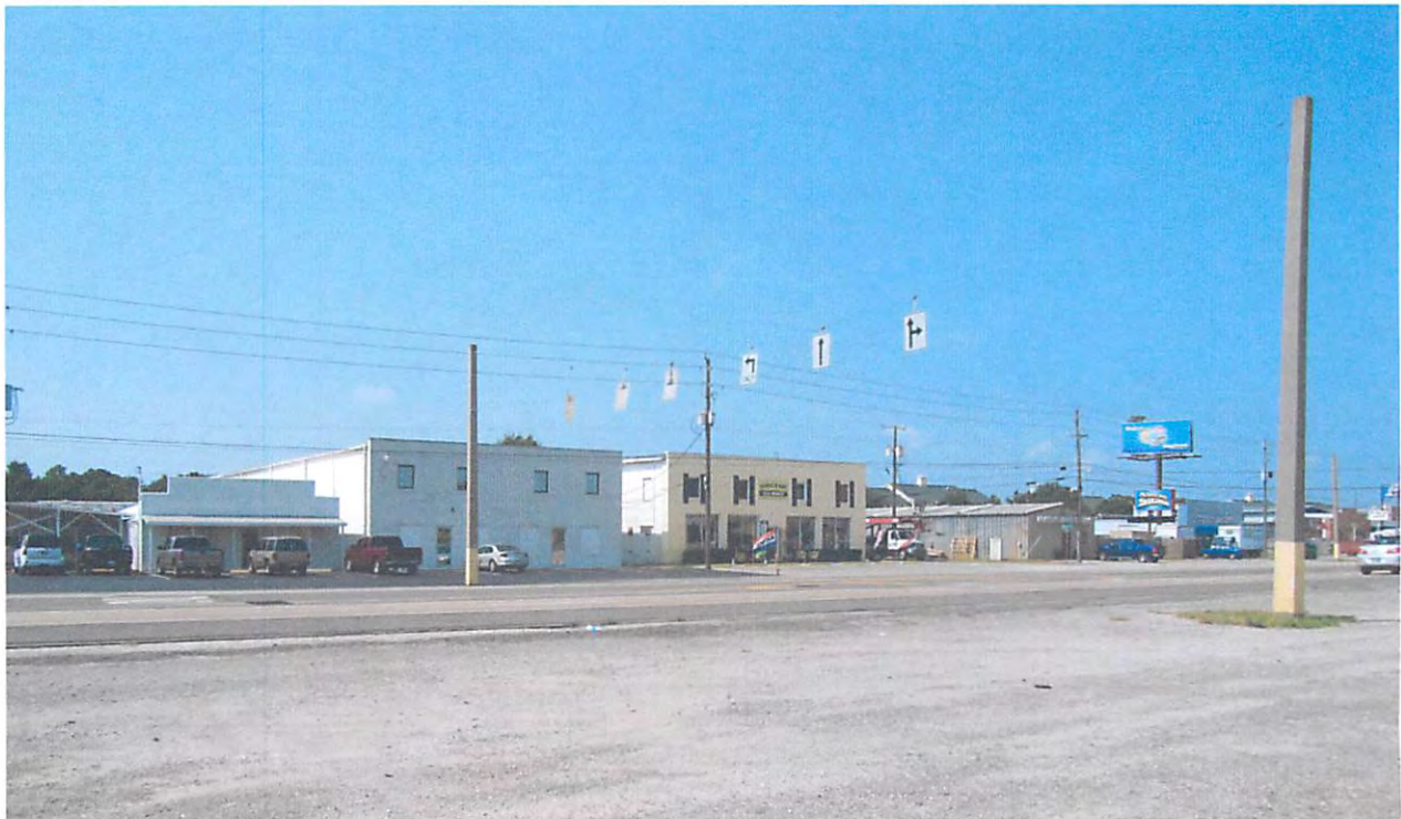
Commercial business located across Navy Blvd
