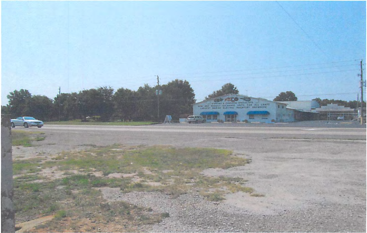
Arco - Marine electric motor repair
